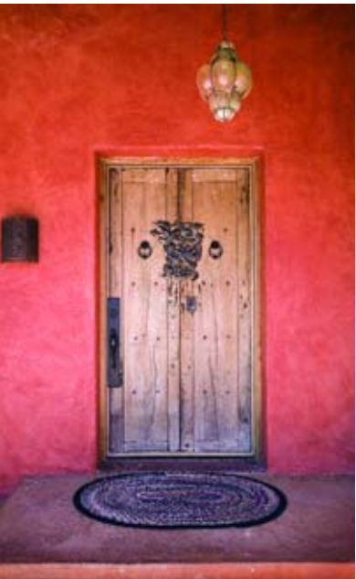
Two old mesquite doors were combined to create the front door.
